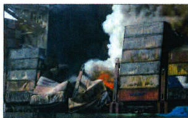
As well as containers on board, the ship's aft and accommodation block were badly damaged in the MAIBAK THORAN incident
