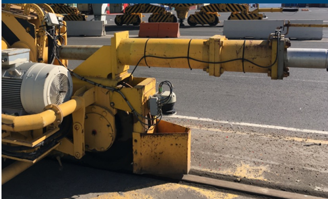
Fig 3: 2D-Laser mounted on the crane
