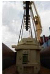
6. Lift commencing with weight of transformer being taken by ship's cranes.
