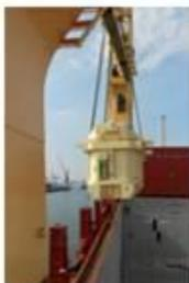
9. Transformer crossing the coaming of the vessel
