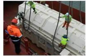
4. Stevedores attaching lifting grommets to lifting points on the transformer
