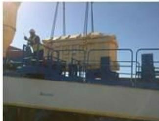
22. Transformer emerging from vessel's hold
