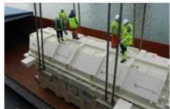
5. Transformer prepared for lifting
