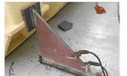
12. Sea fastening completed using 4 x stoppers as shown, attached at the jacking points on transformer
