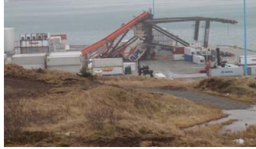
PICTURE: WINDSTORM DAMAGE
