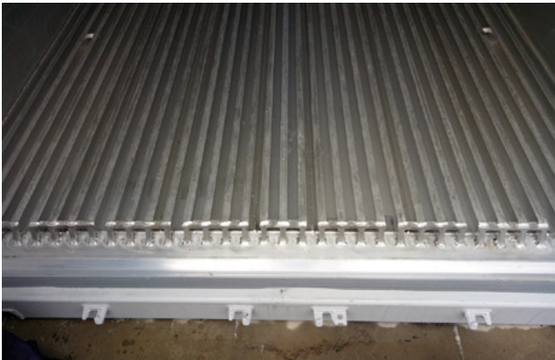
Picture 2 Close up of aluminium T Floor. This is an in-service container with some minor discoloration but otherwise in good condition.
