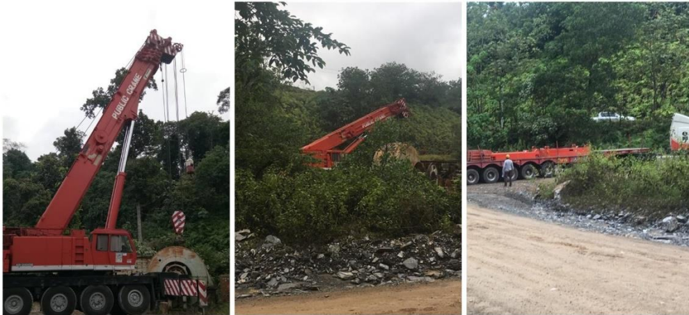
2. Crane, truck and trailer arrival at site.
