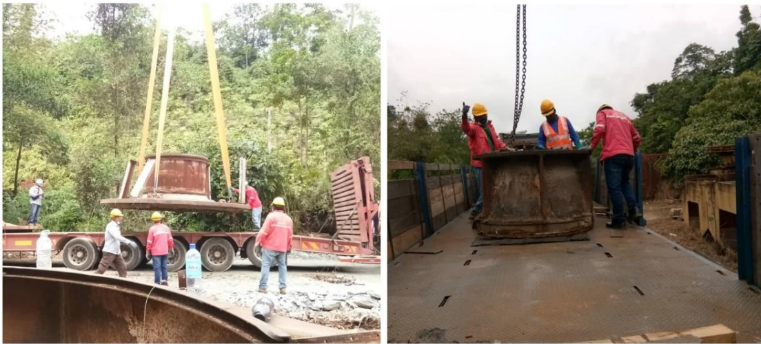
3. Lifting and loading onto the trailers.
