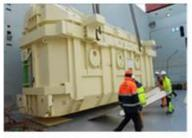
10. Transformer positioned above vessel tanktop; plyboard sheets / dunnage positioned under base of unit
