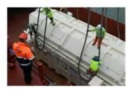
Stevedores attaching lifting grommets to lifting points on the transformer
