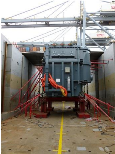
Image: Transformer successfully lashed and secured on the Terra Marique, ready for shipment to the UK
