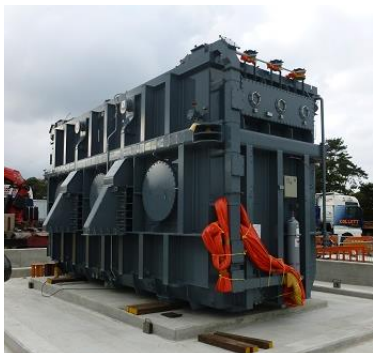
Image 2: Transformer Successfully installed on the Plinth at Sizewell
