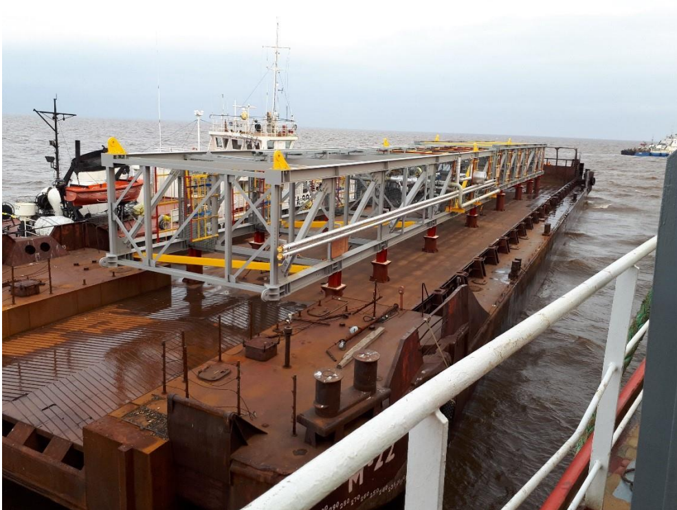
Figure 7. CCR module loaded on a barge
