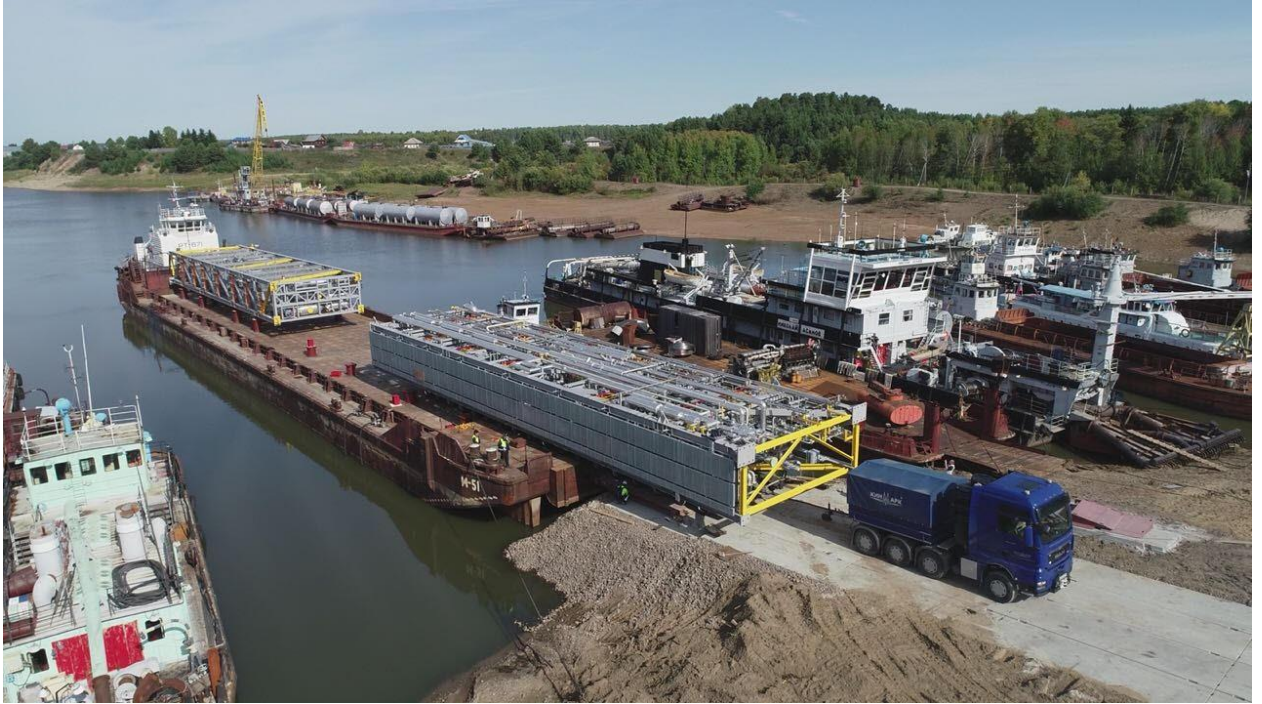
Figure 8. Unloading of CCR module
