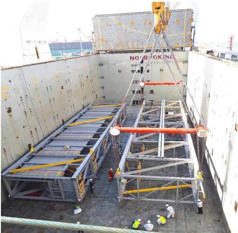
Figure 3. Loading of CCR modules on the sea vessel
